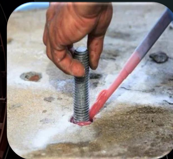
9. Chemical or Adhesive Anchors:
